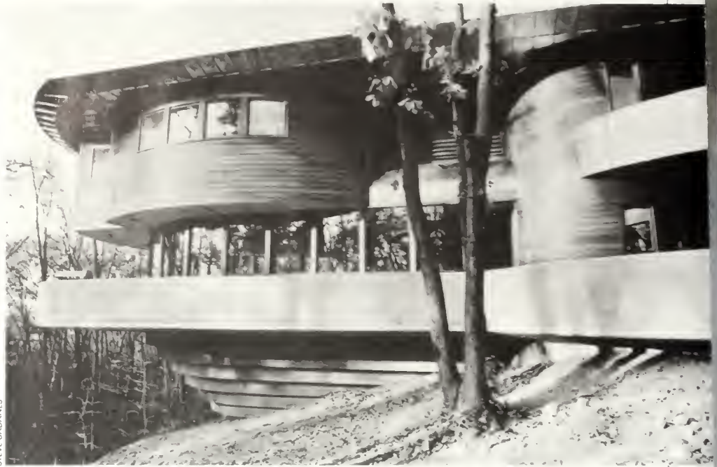
Jutting bowlike, the cantilevered deck from the latest house by the Jersey Devil.
